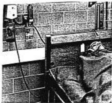
Intermittent vacuum regulator (left) is used in conjunction with piped vacuum system in recovery room.
